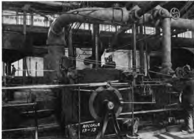
Fig. 2. Operating Device for Governor Bracket, etc.*
